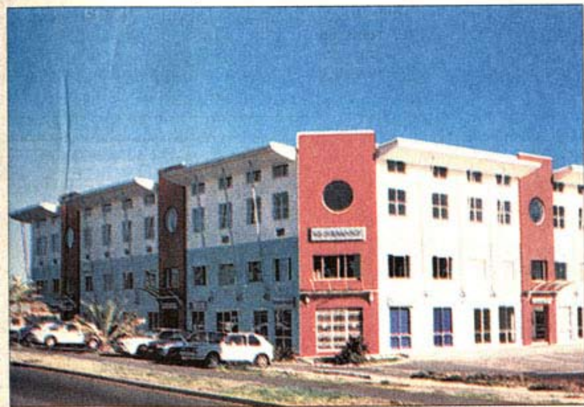
Transformed: 145 on Blaauwberg is a modernised office building
