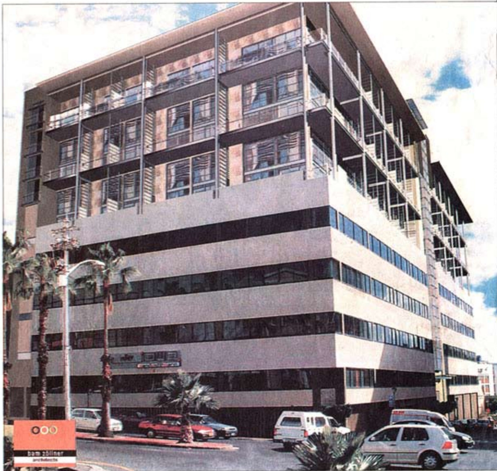
ITS ON TOP: An impression of Soho on Strand to be built on top of the present office block at 128 Strand Street, Cape Town.
