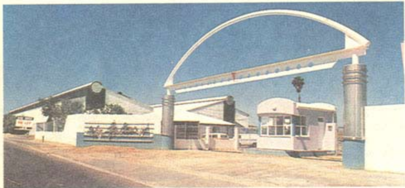
AFTER: The bright new entrance to what is now an industrial park.
